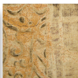
GLW31 Dry Rust
